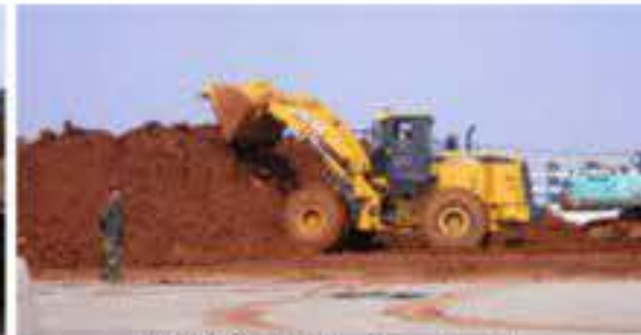
LW800K loader is piling lead zinc ore powder in Panjin port
