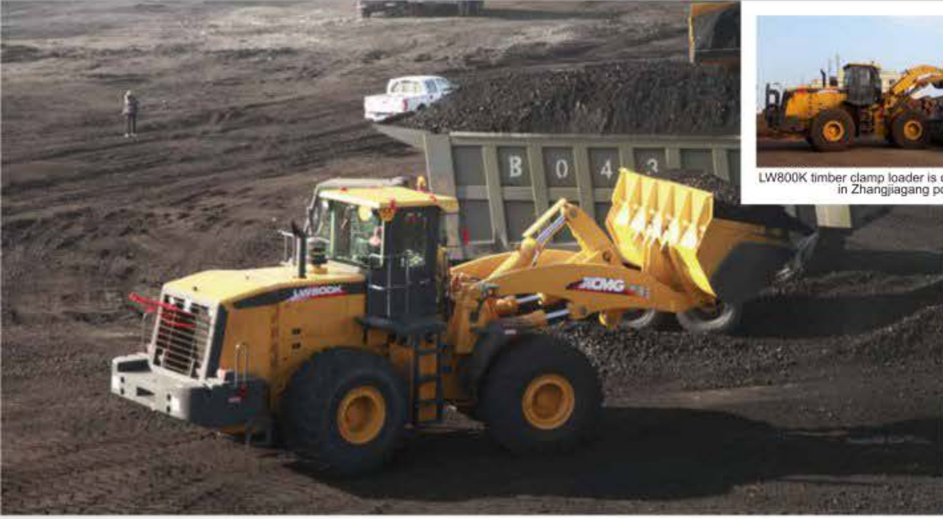
Construction scene of XCMG LW800K loaders
