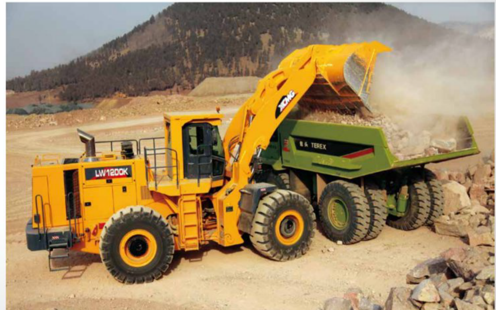
Construction scene of XCMG LW1200K loader, the China's highest tonnage loader
