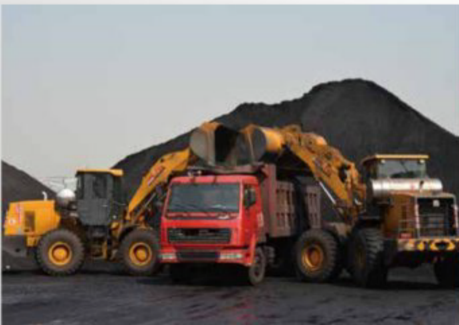
Port construction of XCMG LW500K-LNG loaders
