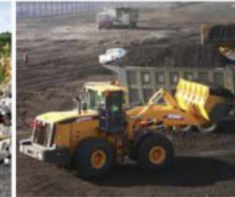
Construction scene of XCMG LW800K loaders
